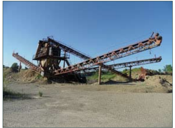
Deister Screening Plant
