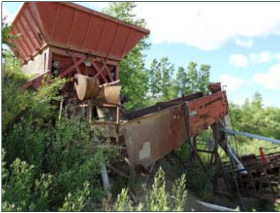
Coarse Material Wash Plant
