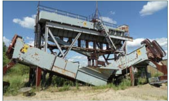
Eagle Iron Works Processing Equip.
