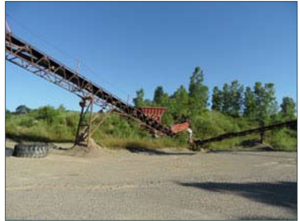
Coarse Material Wash Plant
