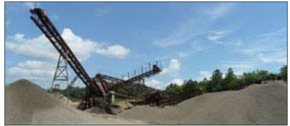
Sand & Gravel Plant
